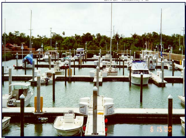
Marina installation of Bellingham Floating Dock System
