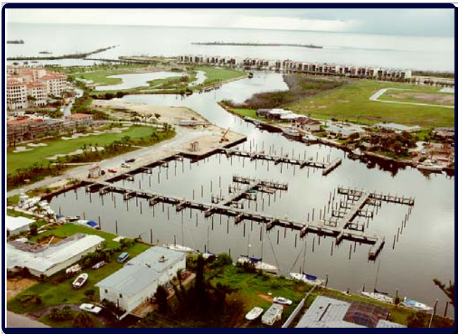
Built ahead of schedule, the Deering Bay Marina in Coral Gables, Florida is one of the many large scale marinas built by our professional construction team.
