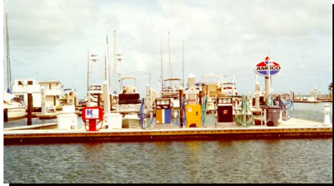
Providing the ultimate in design flexibility. Floating fuel facilities can be located almost anywhere within the boundaries of the marina.
